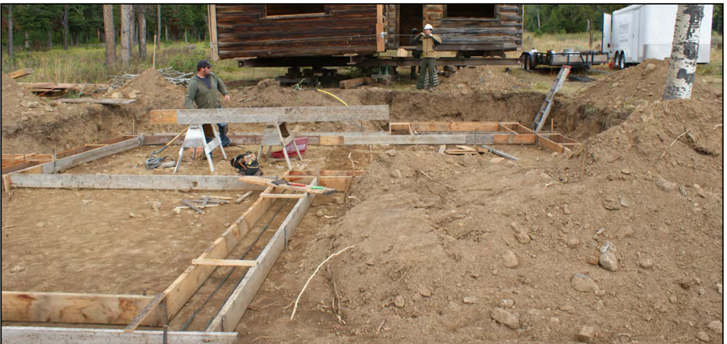
Deteriorated sill logs were replaced in kind, and the cabin stabilized before work began. In fall of 2010, the cabin was lifted, the existing foundation removed and a new foundation was poured.
