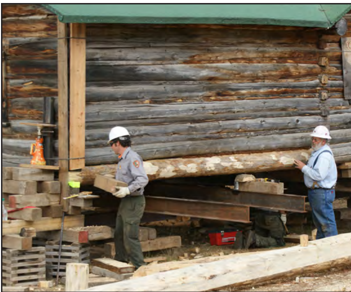
Deteriorated sill logs were replaced in kind, and the cabin stabilized before work began. In fall of 2010, the cabin was lifted, the existing foundation removed and a new foundation was poured.
