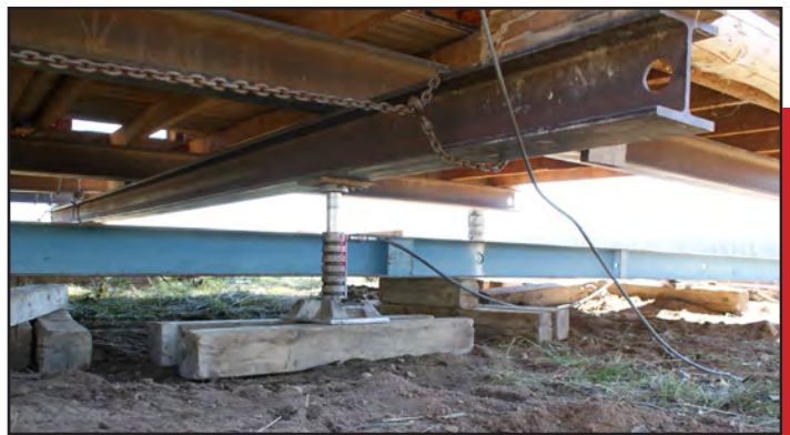
Deteriorated sill logs were replaced in kind, and the cabin stabilized before work began. In fall of 2010, the cabin was lifted, the existing foundation removed and a new foundation was poured.
