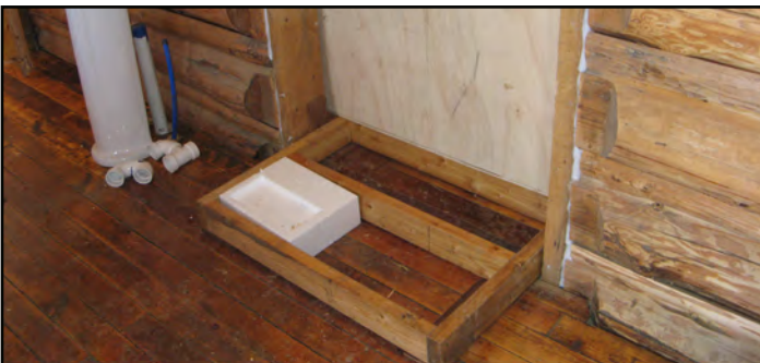
The door opening between rooms was closed off and used as as a built in shelving space.
