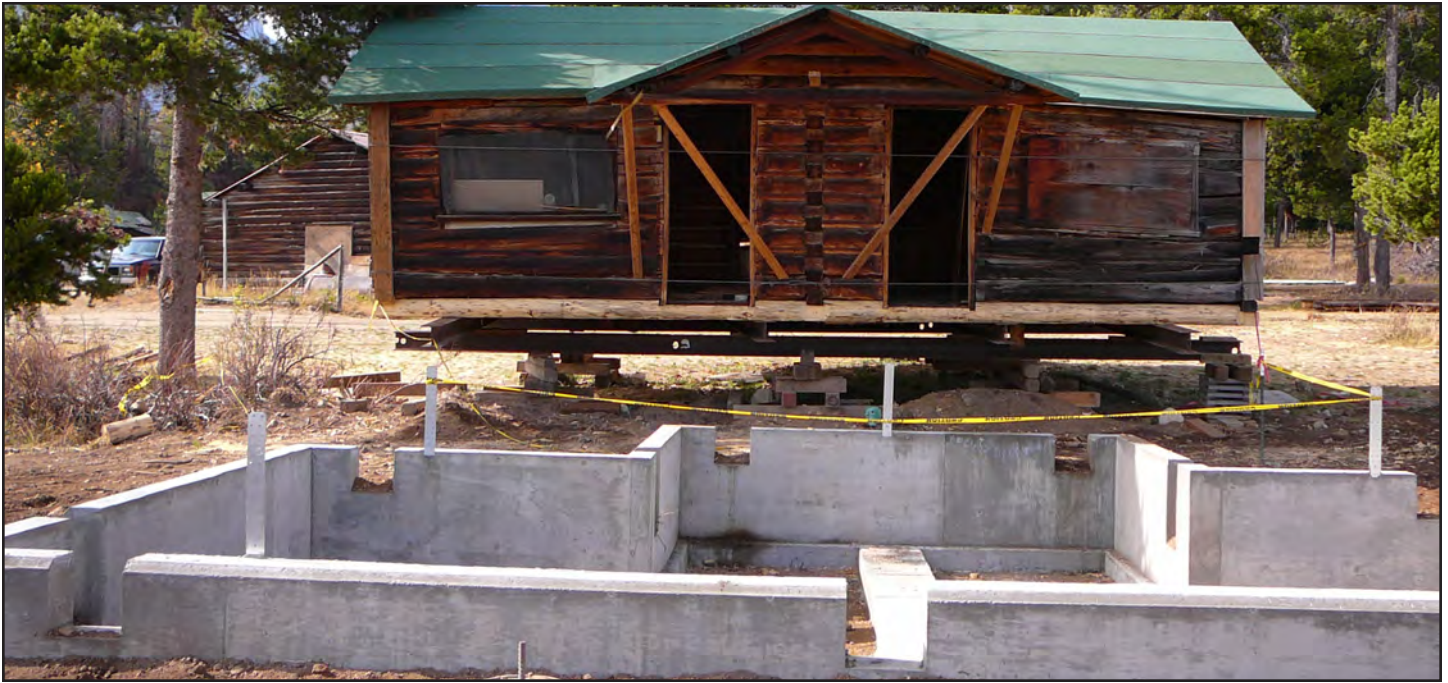
Below: New concrete foundation before cabin is moved back in place.
