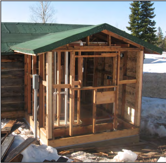
Below: Work on the bathroom addition, spring, 2011
