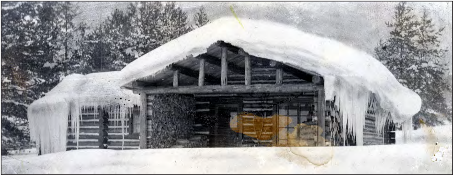
Above: Hammond Cabin, circa 1925, prior to additions. Photo courtesy of the Gale family.
