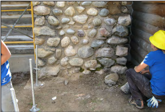
Both fireplaces had loose stones at the top of the chimneys and deteriorating mortar that was repaired with help from our Student Conservation Association (SCA) masonry team.
