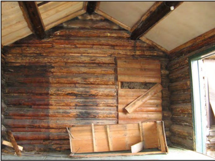
Pictured: Initial photos taken in 2006, and 2007 before preservation efforts began.
