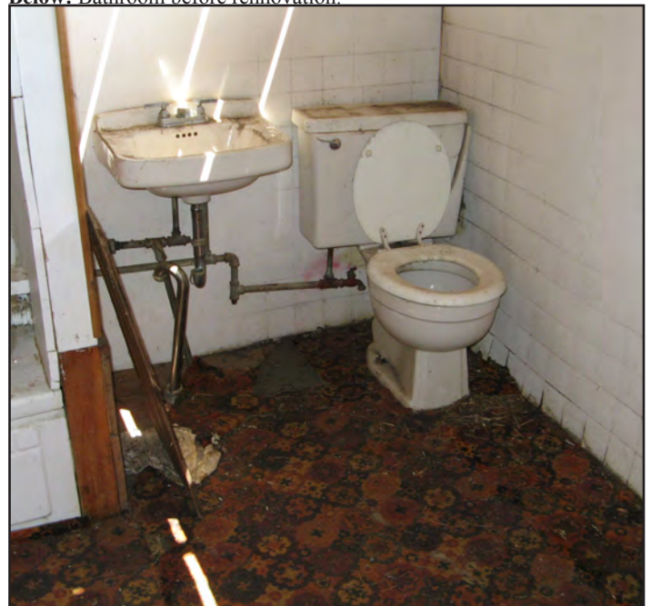
Below: Bathroom before renovation.
