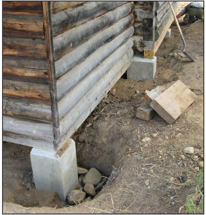
The rotted flooring was taken out, and the cabin was reset on new concrete foundations (including a crawl space). Deteriorated sill and wall logs were all replaced in-kind.
