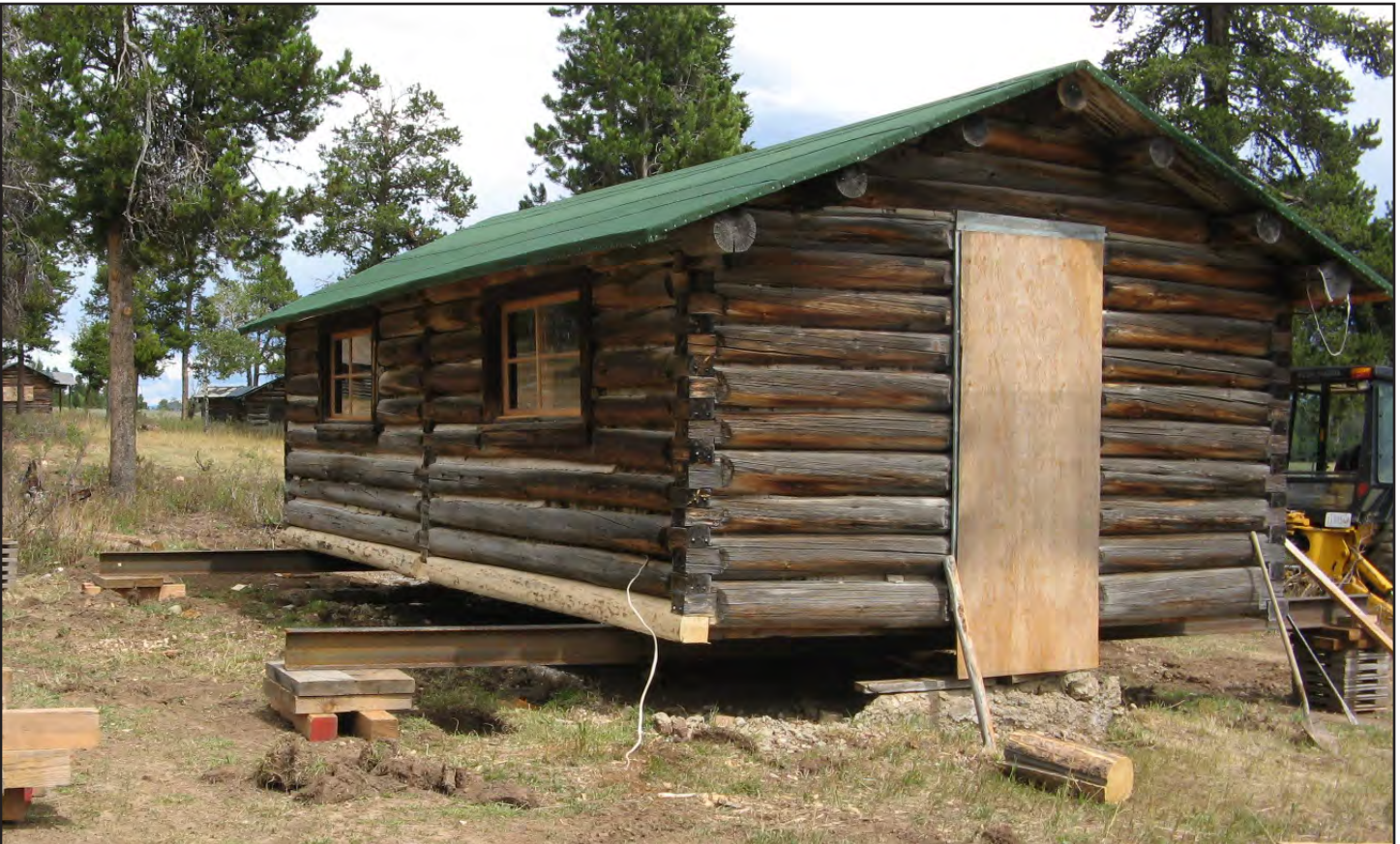
The rotted flooring was taken out, and the cabin was reset on new concrete foundations (including a crawl space). Deteriorated sill and wall logs were all replaced in-kind.
