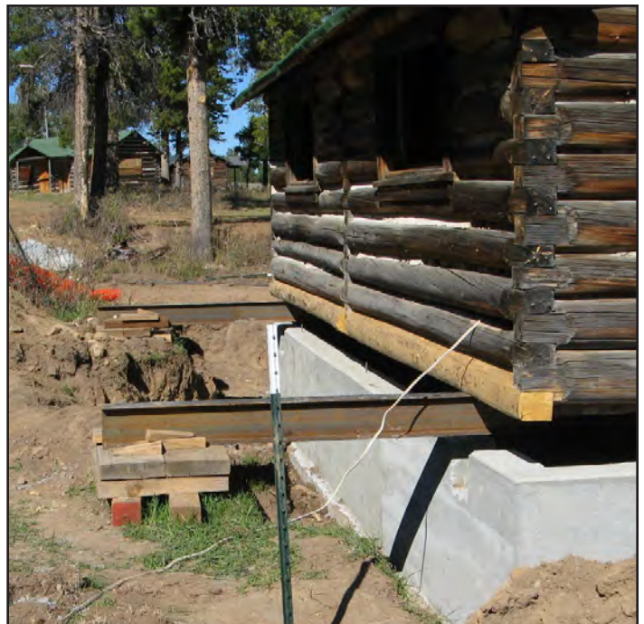
2009: The cabin was lifted, the existing foundation removed and a new foundation was poured.
