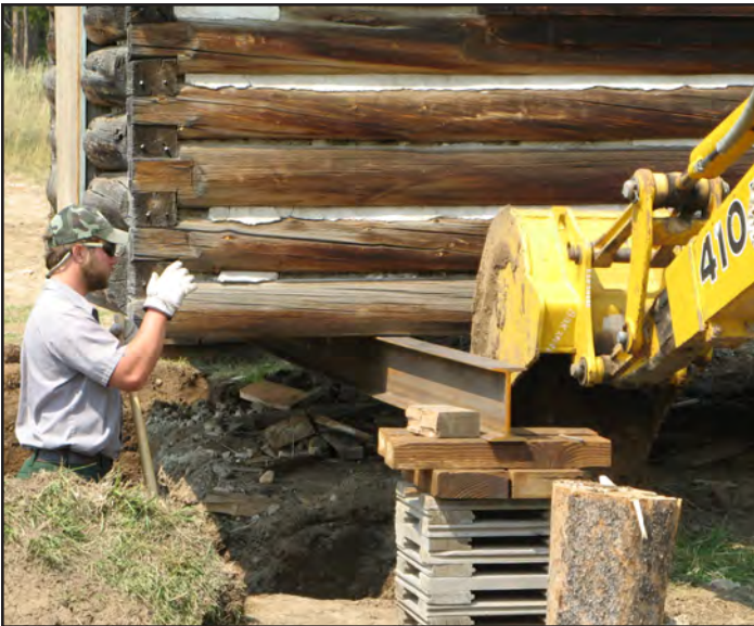
2009: The cabin was lifted, the existing foundation removed and a new foundation was poured.
