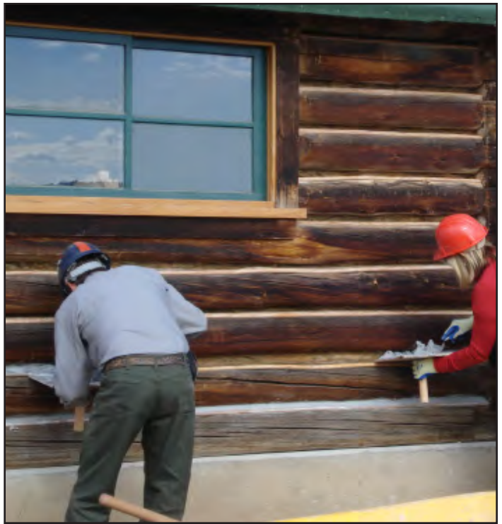
Windows and doors were treated at the WCHP shop in Moose while replacing cabin logs in-kind. New exterior chinking was done with help from volunteers in 2008.
