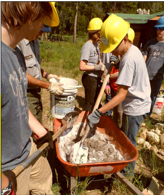
Above: Becket Chimney Corner volunteers mix the daubing material in a wheelbarrow, 2013.
