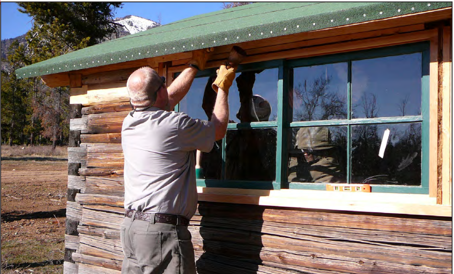
Windows and doors were treated at the WCHP shop in Moose while replacing cabin logs in-kind. New exterior chinking was done with help from volunteers in 2008.
