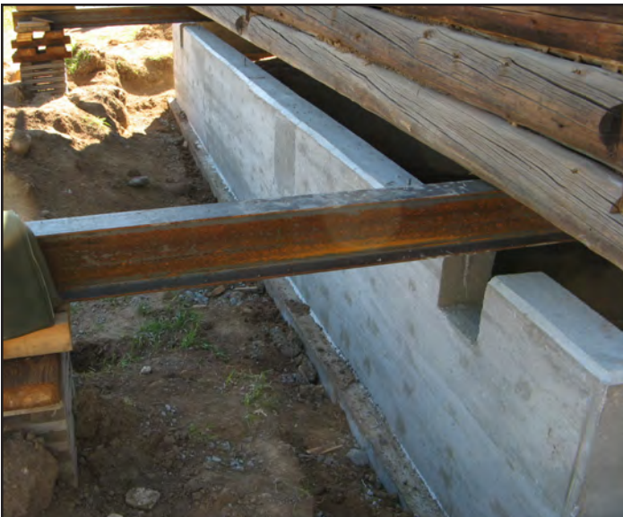
2009: The cabin was lifted, the existing foundation removed and a new foundation was poured.
