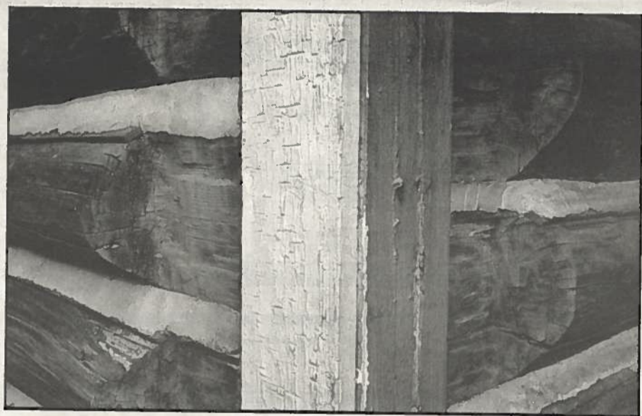
The old Van Vleck house (a.k.a. Jedediah's House of Sourdough) sports corners that were cut and squared by axe and peeled with a draw knife.
