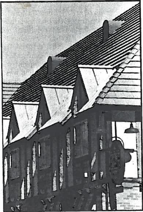
The Wort Hotel is one site that could be on the National Historic Register listing.
