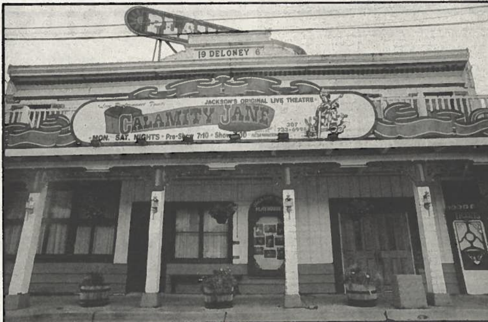
The Jackson Hole Playhouse is said to be the oldest building in town on its original site. Only town regulation would ensure its preservation.
