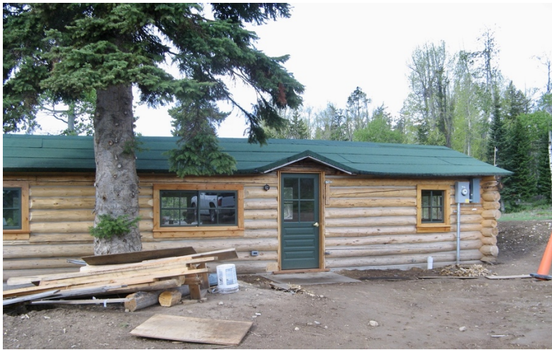
New wall under construction while the historic tree remained intact, 2012.
