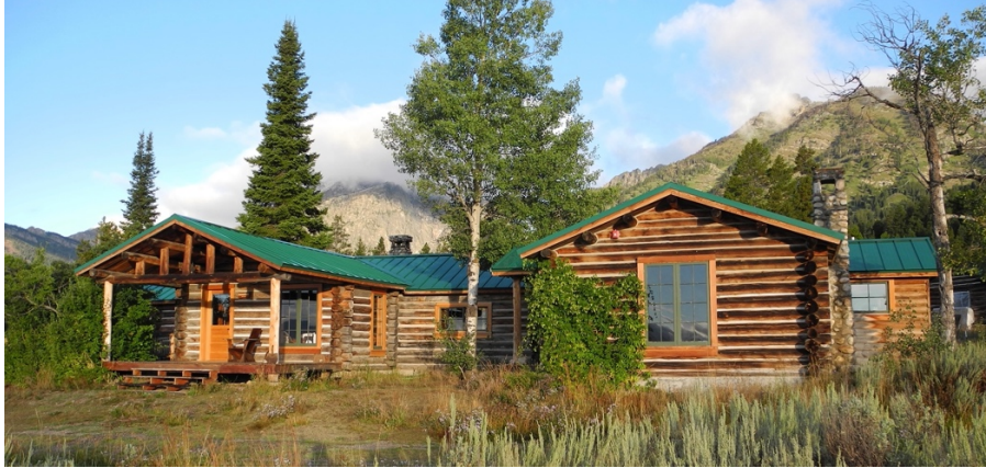
Rehabilitated Hammond Cabin containing conference room, kitchen, storage room and caretaker's quarters.
