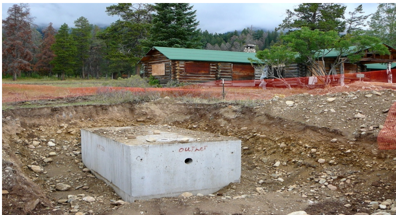
Installing new sewer system in front of the Hammond Cabin, 2007.
