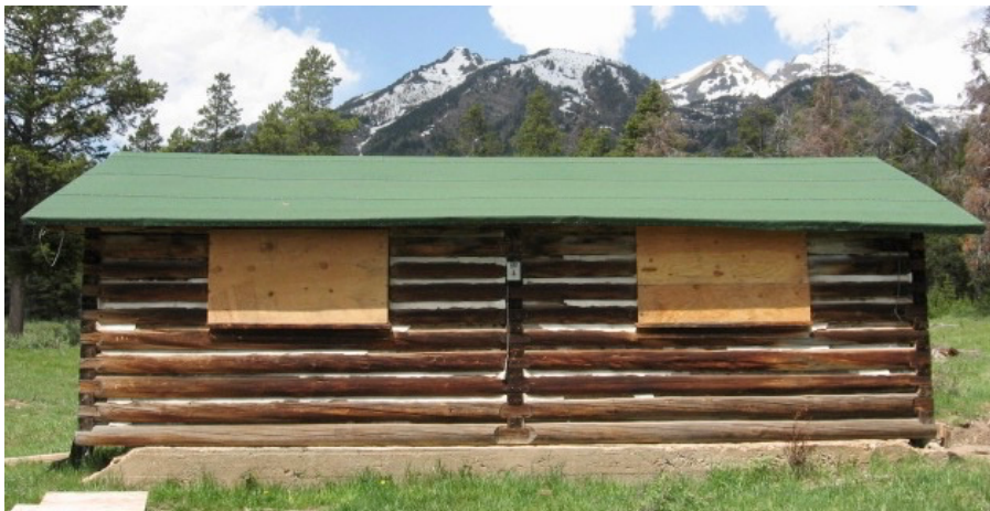
Example of traditional rolled roofing; life expectancy in White Grass environment is about 8 years.
