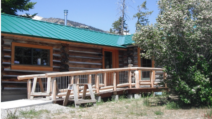
Metal roof on Hammond Cabin, 2012.
