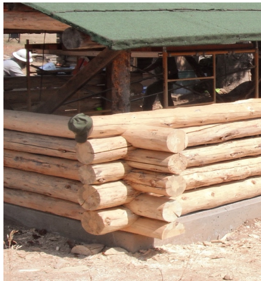
Much more stable saddle notch corners, Main Cabin, 2012.
