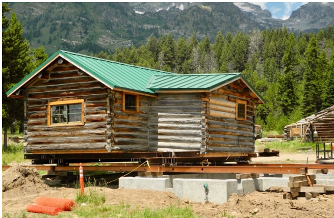
Cabin 1161 being moved back onto a new foundation, circa 2014.
