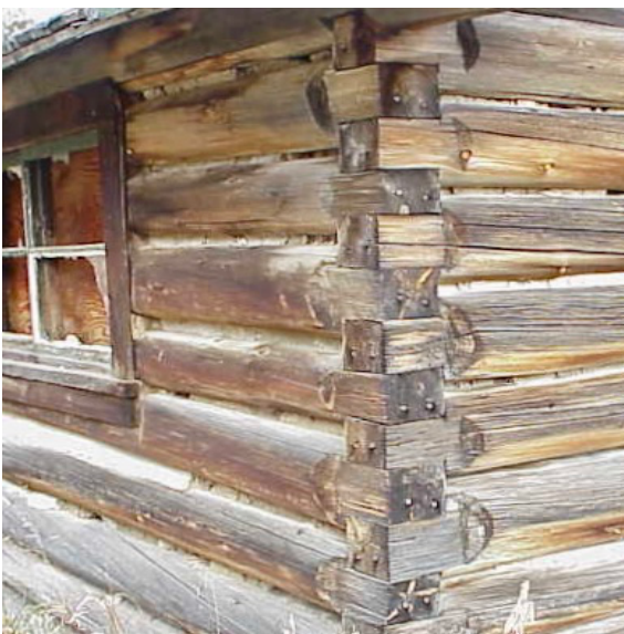
Example of hog trough corners.
