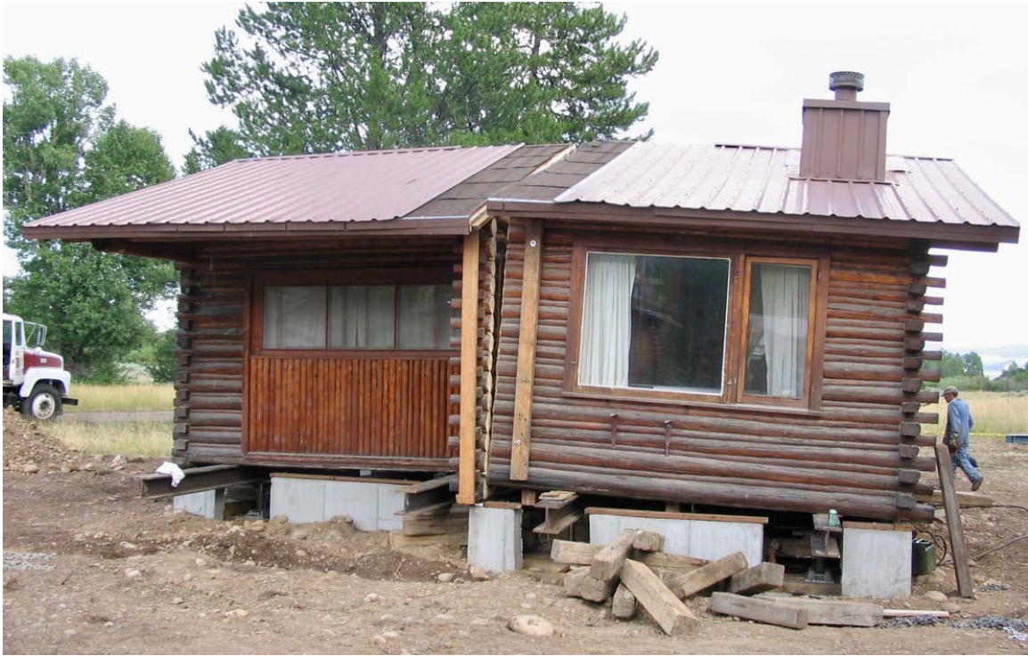
To prepare this cabin for transport, it was cut in half while at the JY Ranch. Once relocated to Beaver Creek, the two halves were merged and placed on a new foundation. Photo courtesy of WCHP, 2005.
