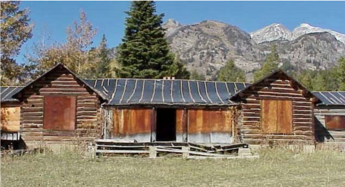
Pre-rehabilitation of White Grass Ranch Main Cabin. Photo courtesy of WCHP, 2013.
