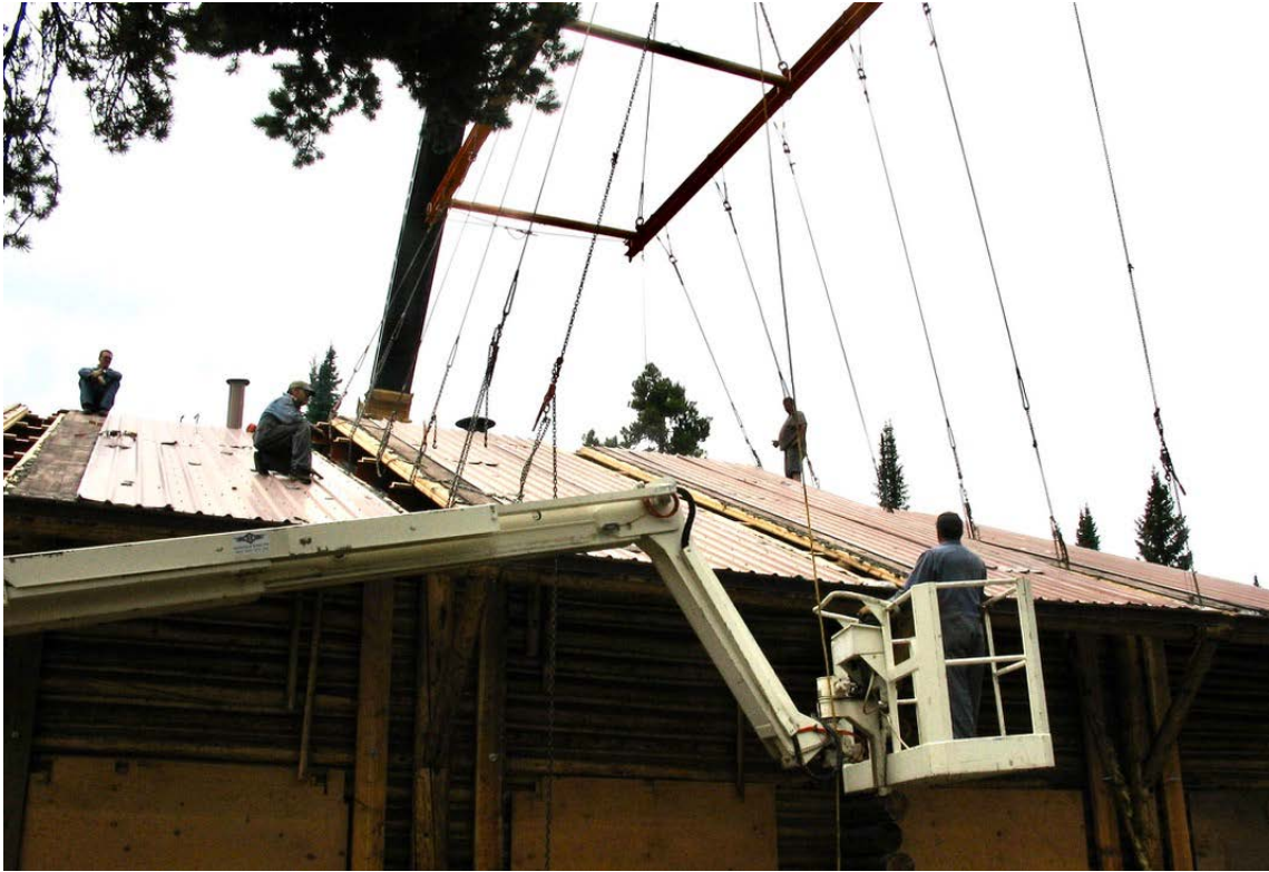
Beginning the process of dismantling the roof. Photo courtesy of WCCP, 2005.
