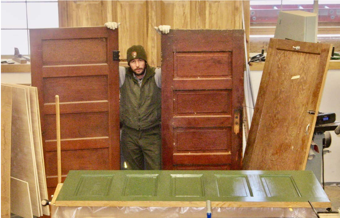
Doors repaired/rebuilt and new doors duplicated in Moose Shop. Photo courtesy of WCHP, 2011.
