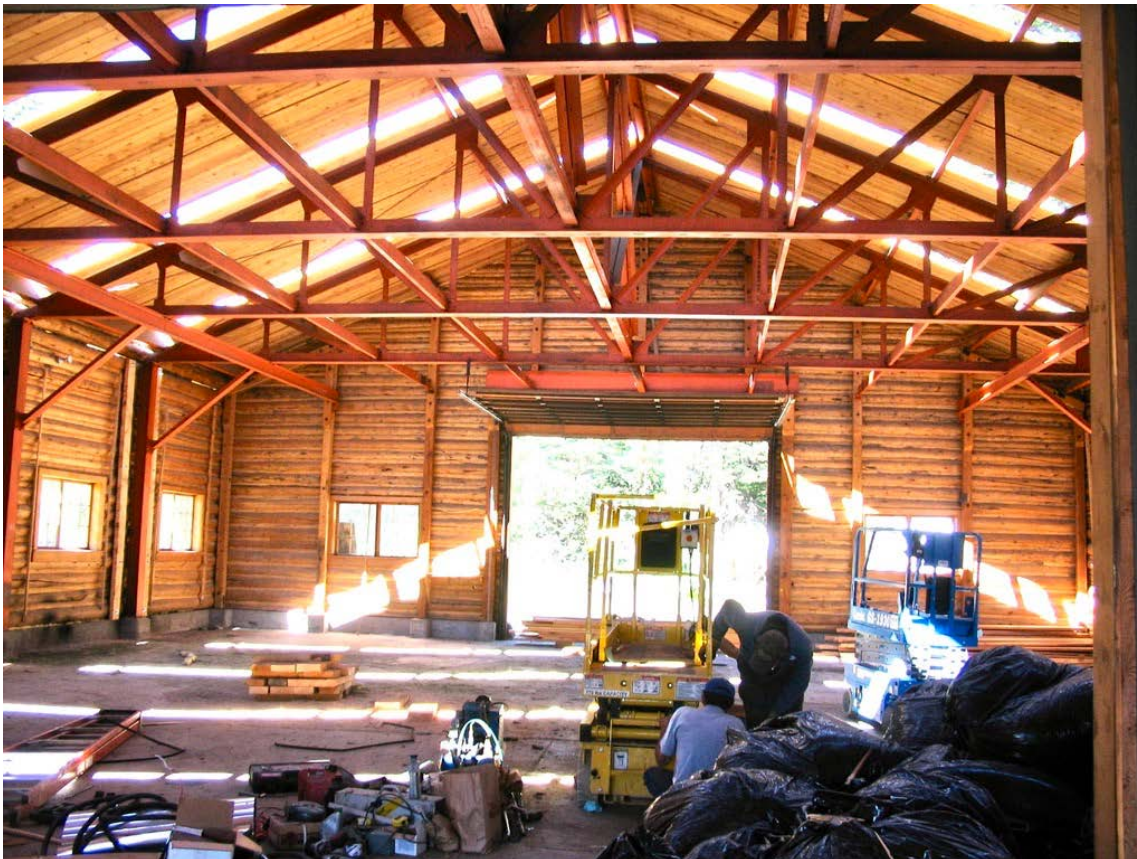
Steel structure inside the JY Shop. Photo courtesy of WCCP, 2005.
