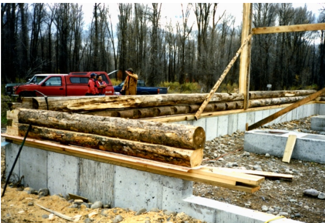
Reassembling White Grass Barn using many original barn logs. Photo courtesy of Carole Hofley.
