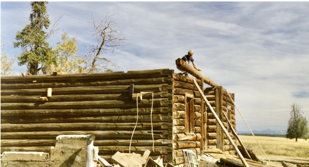
Lowering the logs with ropes. Photo courtesy of Cavicchioni & Gerster.
