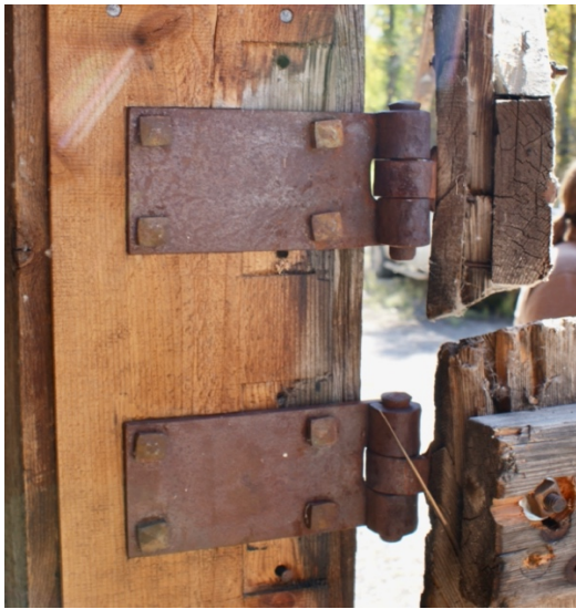
Hand forged hardware on the entrance doors to the barn. Photo courtesy of Craig Struble.
