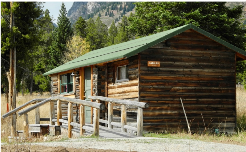
Cabin 1155 with ADA accommodations, 2012. Photo courtesy of R. Butterbaugh.
