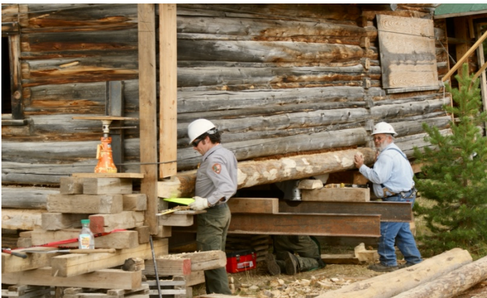
Chris Frank (L) and Jack Shinkle (R) replace a log on Cabin 1161. Photo Courtesy of R. Butterbaugh, 2011.
