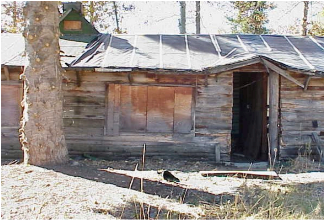
Kitchen Pre-rehabilitation, 2010. Photo courtesy of WCHP.
