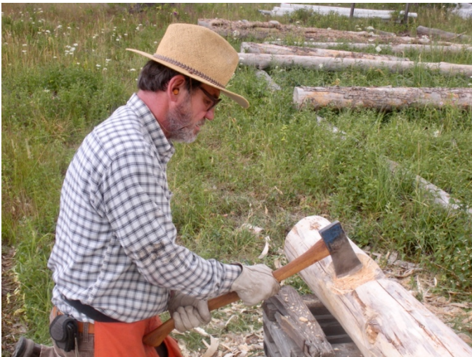
Creating a saddle notch in a log for the Main Cabin Kitchen with an axe, 2013. Photo courtesy of R. Butterbaugh.
