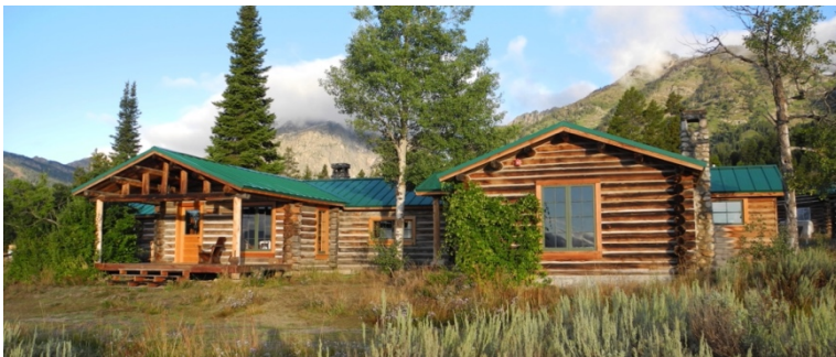
Completed Hammond Cabin. Photo courtesy of R. Butterbaugh, 2011.
