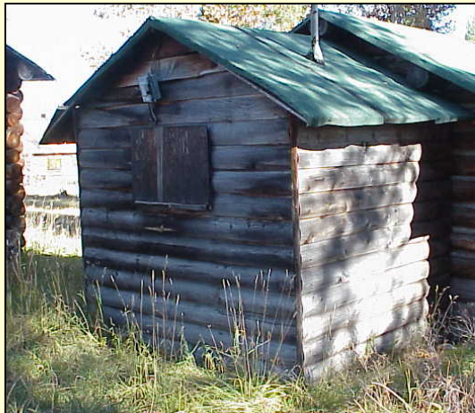
repair bathroom additions
