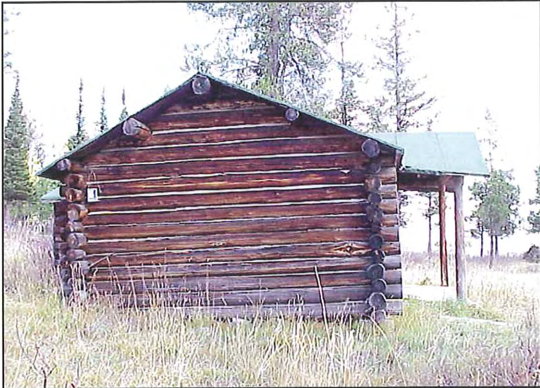
Figure 74. South wall of HS-1163, Cabin 7. Source: A&E Architects, 2004.
