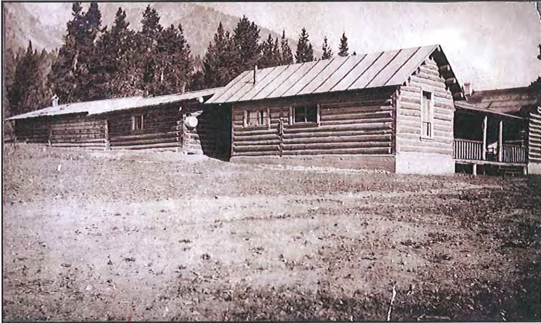
Figure 4. Circa 1925 photograph of the south and east walls of the building known during the dude ranch era as the Main Cabin, HS-1168. This is believed to be Harold Hammond's original homestead house. Photo courtesy of Frank Galey's family.
