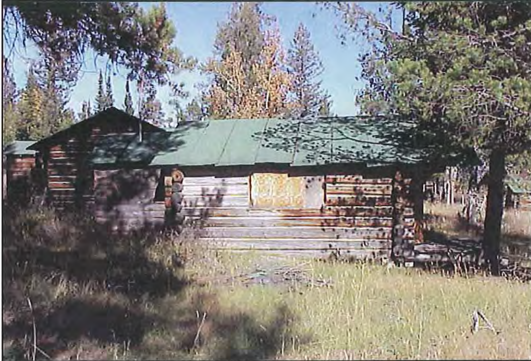
Figure 86. South wall of HS-1165, Cabin 5. Source: A&E Architects, 2004.
