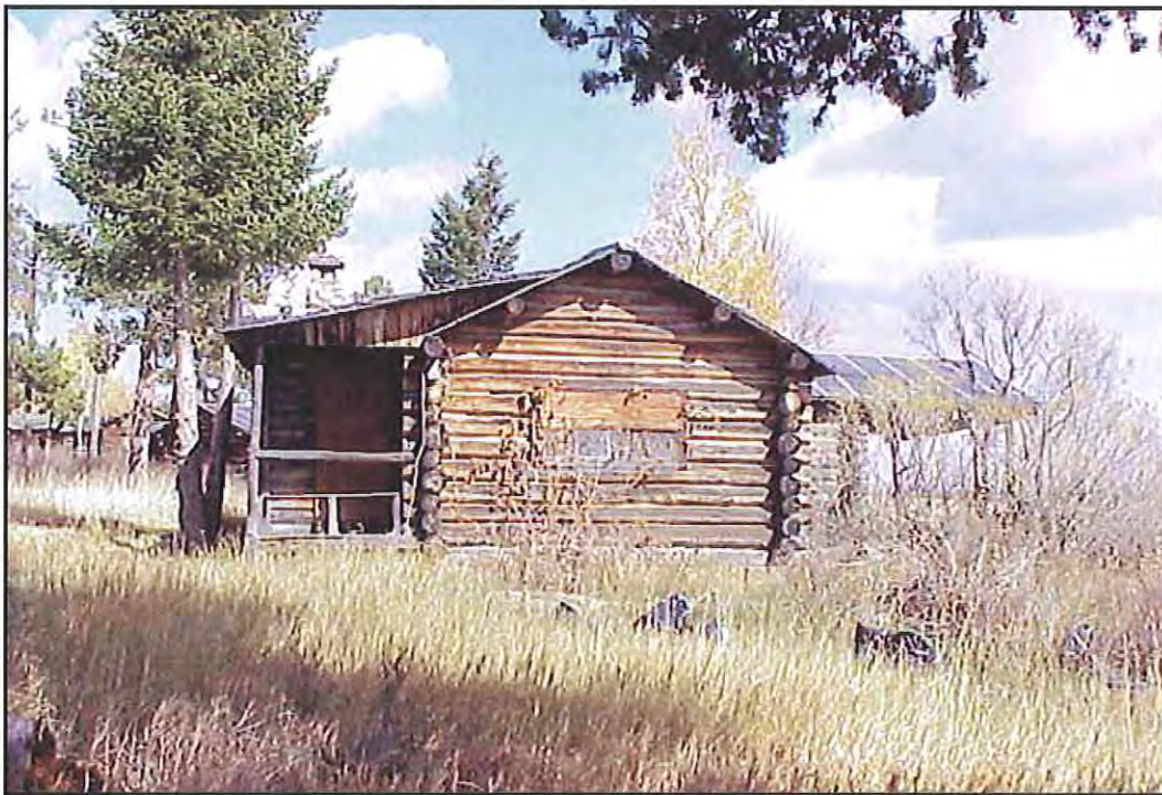
Figure 33. South wall of HS-1156, Hammond Cabin. Source: A&E Architects, 2004.
