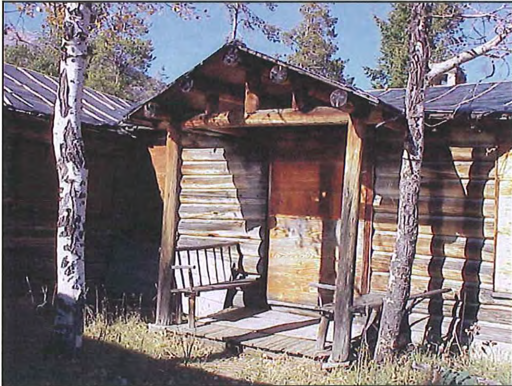
Figure 34. Exterior porch on south wall of north addition, HS-1156, Hammond Cabin. Source: A&E Architects, 2004.
