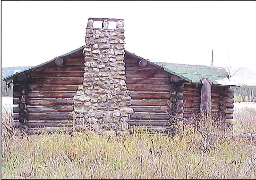
Figure 52. West wall of HS-1159, Cabin 9. Source: A&E Architects, 2004.
