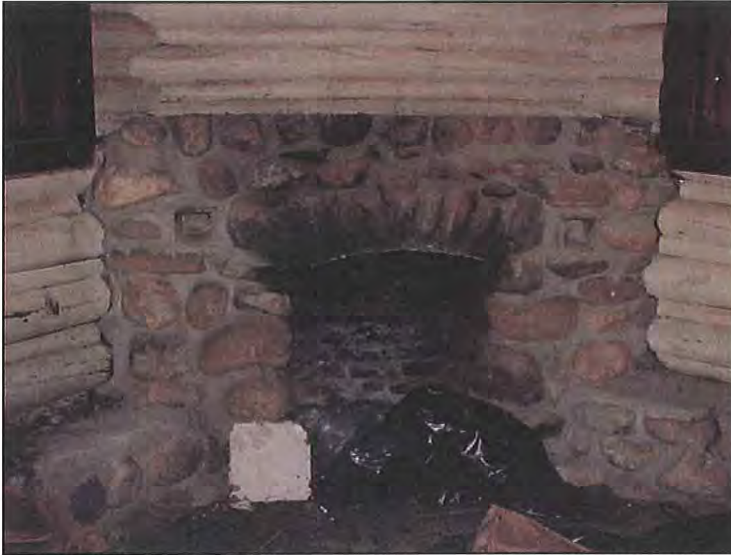
Figure 93. Interior fireplace with stone seats in the card room, north end of HS-1168, the Main Cabin. Source: A&E Architects, 2004.
