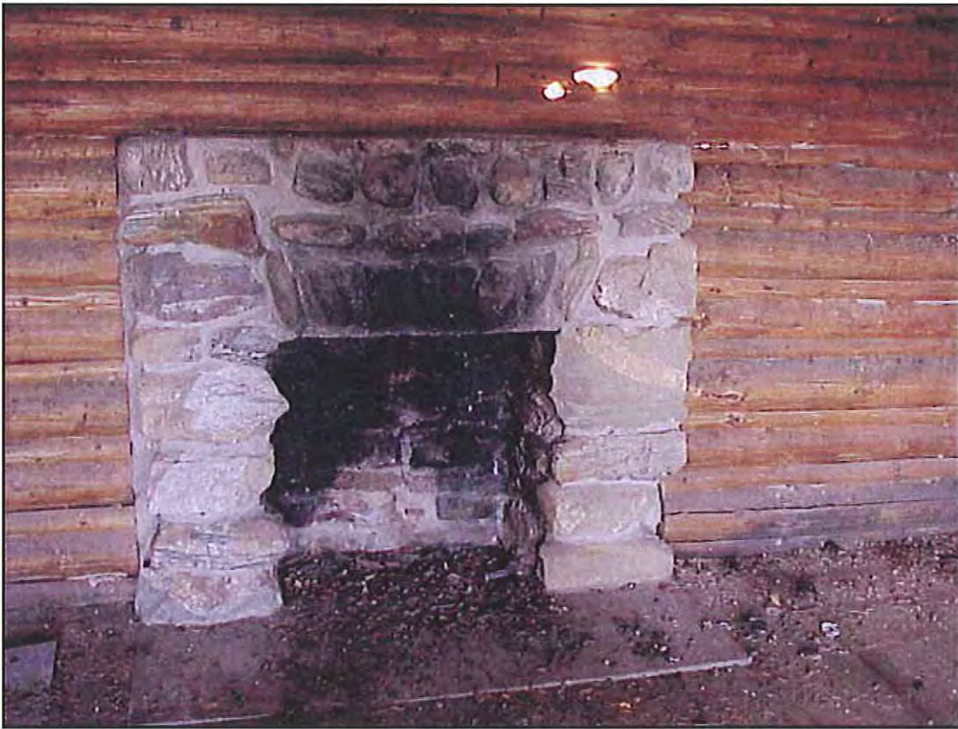
Figure 53. Interior fireplace, rear (west) wall of HS-1159, Cabin 9. Source: A&E Architects, 2004.
