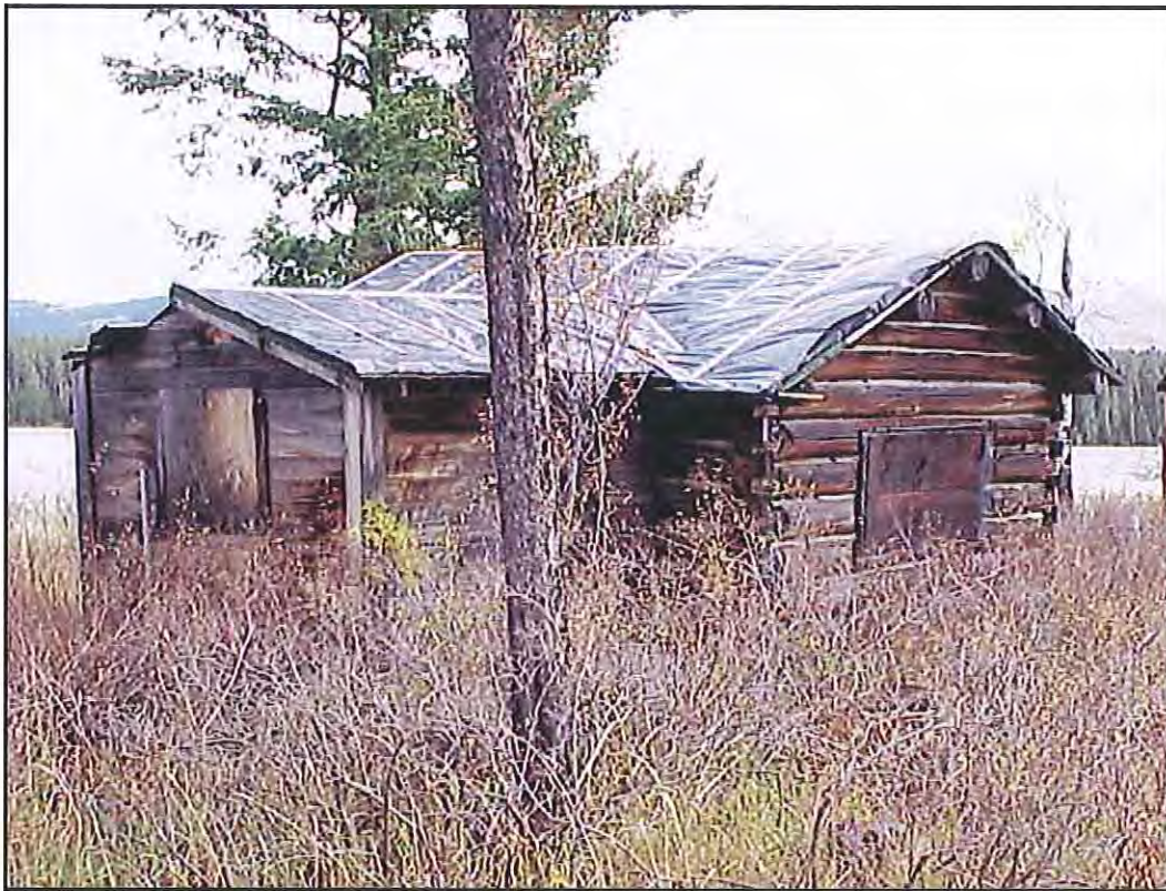
Figure 40. North and west walls of HS-1157, Cabin 12. Source: A&E Architects, 2004.
