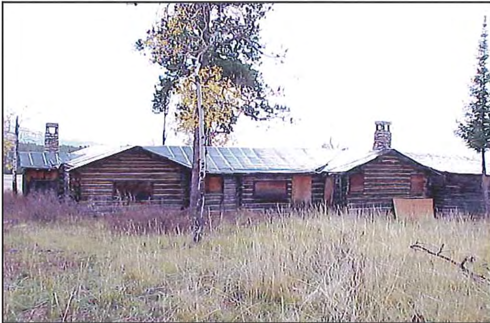
Figure 31. West wall of HS-1156, Hammond Cabin. Source: A&E Architects, 2004.
