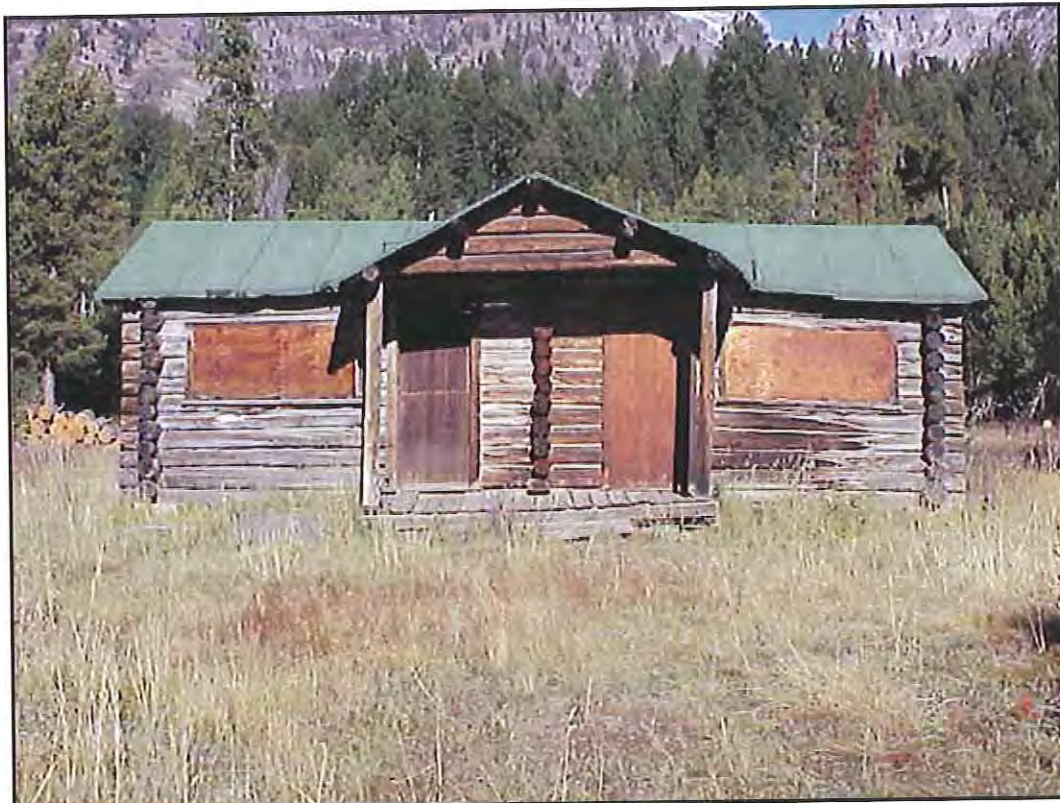
Figure 71. East (front) wall of HS-1163, Cabin 7. Source: A&E Architects, 2004.
