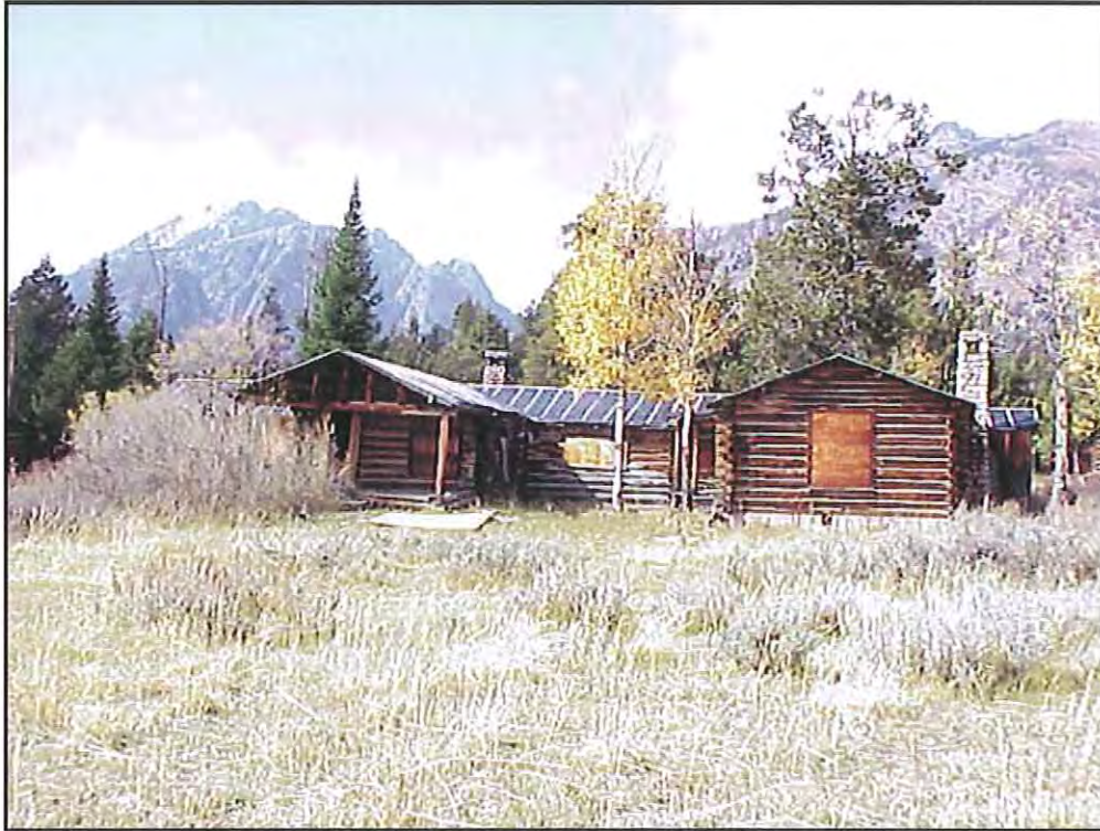
Figure 30. Front (east) wall of HS-1156, Hammond Cabin. The open porch visible at the south end of the building is part of the original building. Everything north of the porch is an addition. Source: A&E Architects, 2004.
