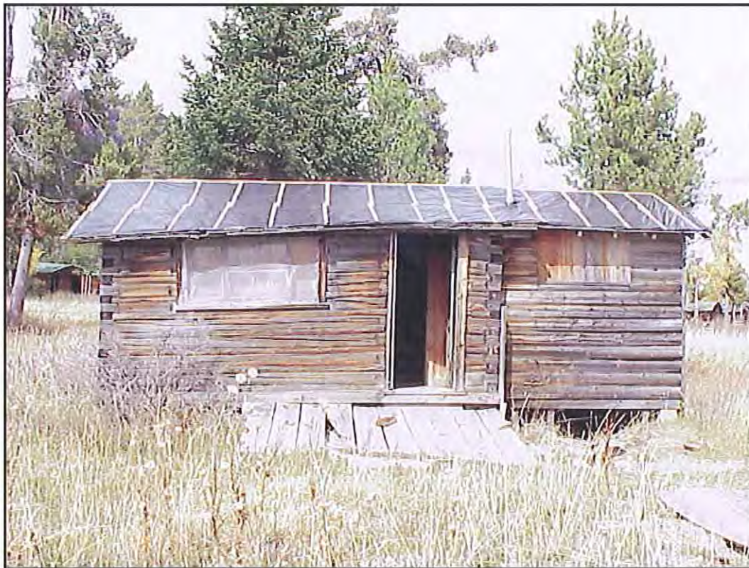
Figure 25. South wall of HS-1155, Cabin 15; bathroom addition to right. Source: A&E Architects, 2004.
