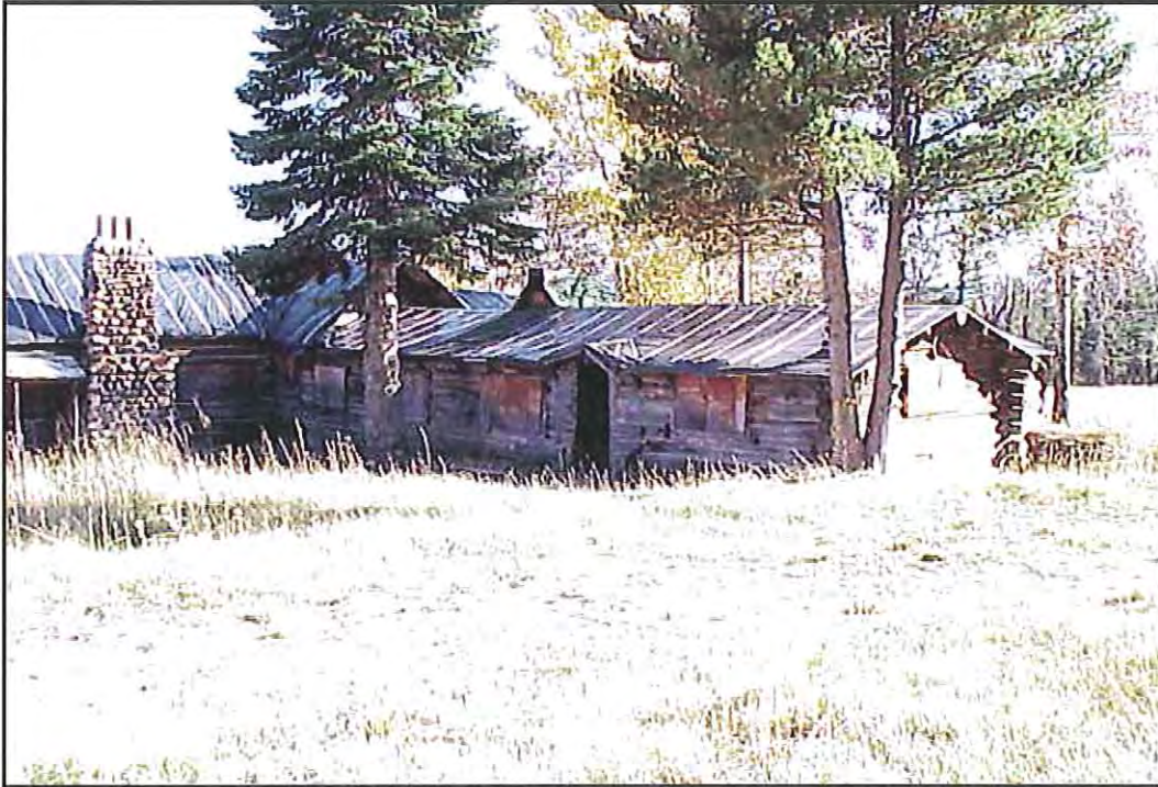
Figure 91. North and west walls of the west wing, HS-1168, the Main Cabin. Source: A&E Architects, 2004.
