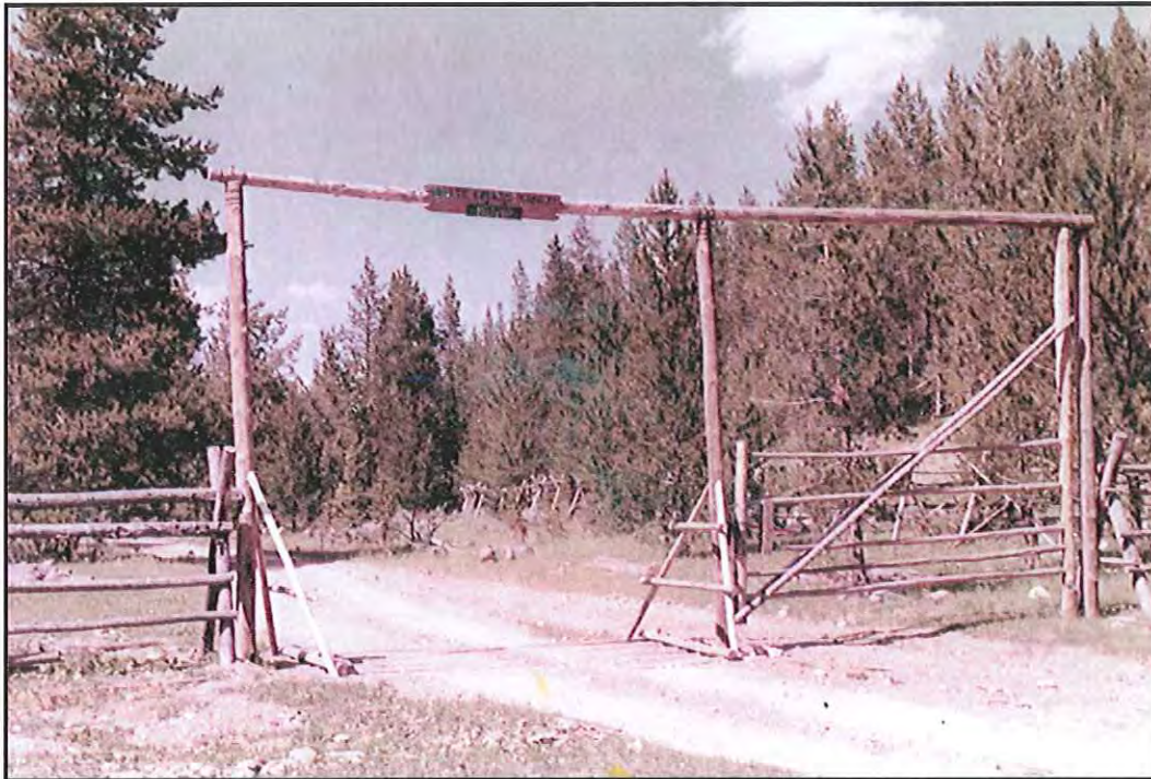
Figure 118. Photograph of the entrance gate to White Grass Ranch, circa 1965. This gate was located at the south end of the main road, just north of its junction with the Death Canyon road. Photo courtesy of Frank Galey's family
