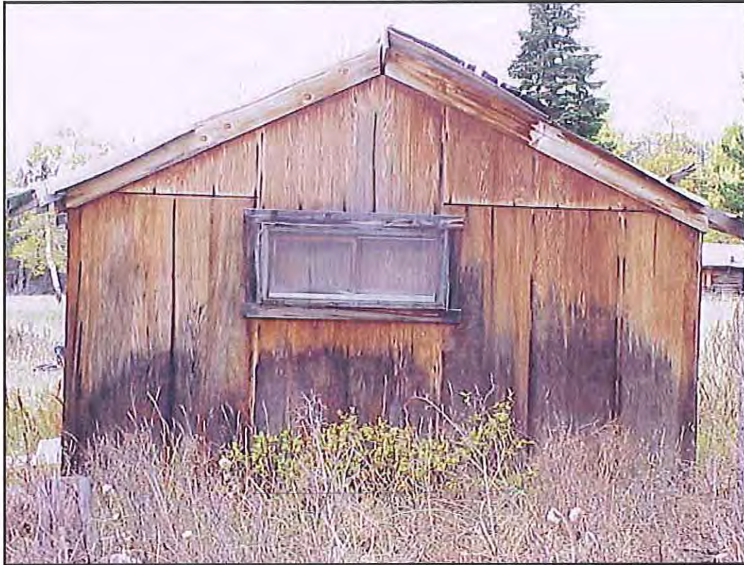
Figure 23. North wall of the addition HS-1154, Girls' Cabin. Source: A&E Architects, 2004.
