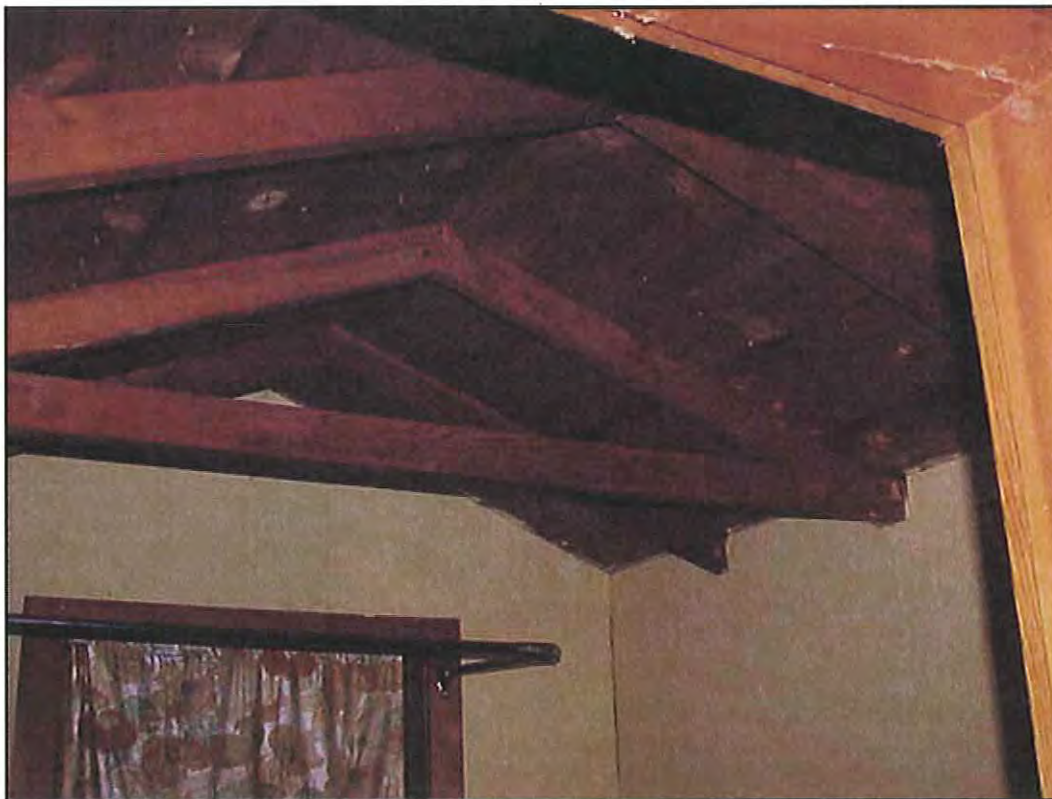
Figure 81. Interior of the bathroom addition in HS-1164, Cabin 6. Source: A&E Architects, 2004.
