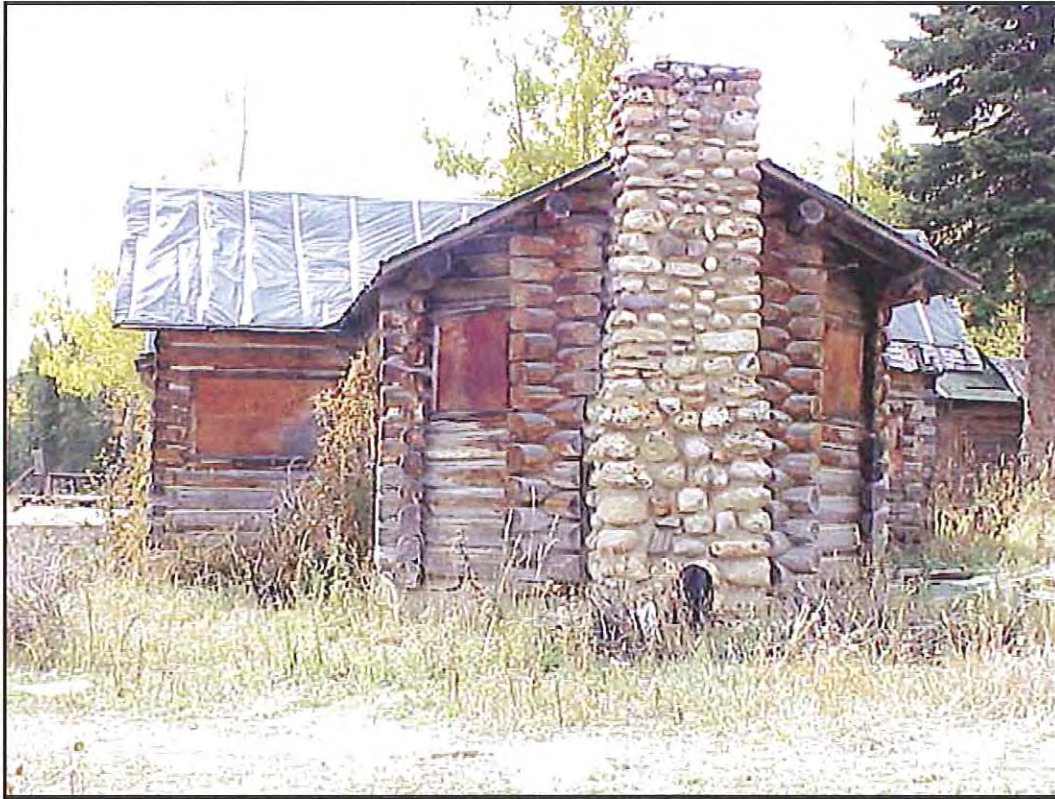
Figure 89. North wall of HS-1168, the Main Cabin. Source: A&E Architects, 2004.
