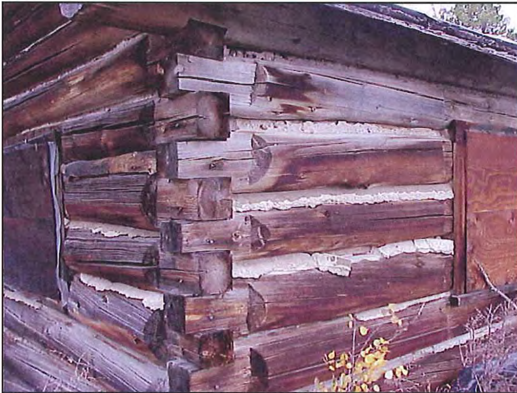
Figure 42. Detail of the corner notching and wall daubing in HS-1157, Cabin 12. Source: A&E Architects, 2004.
