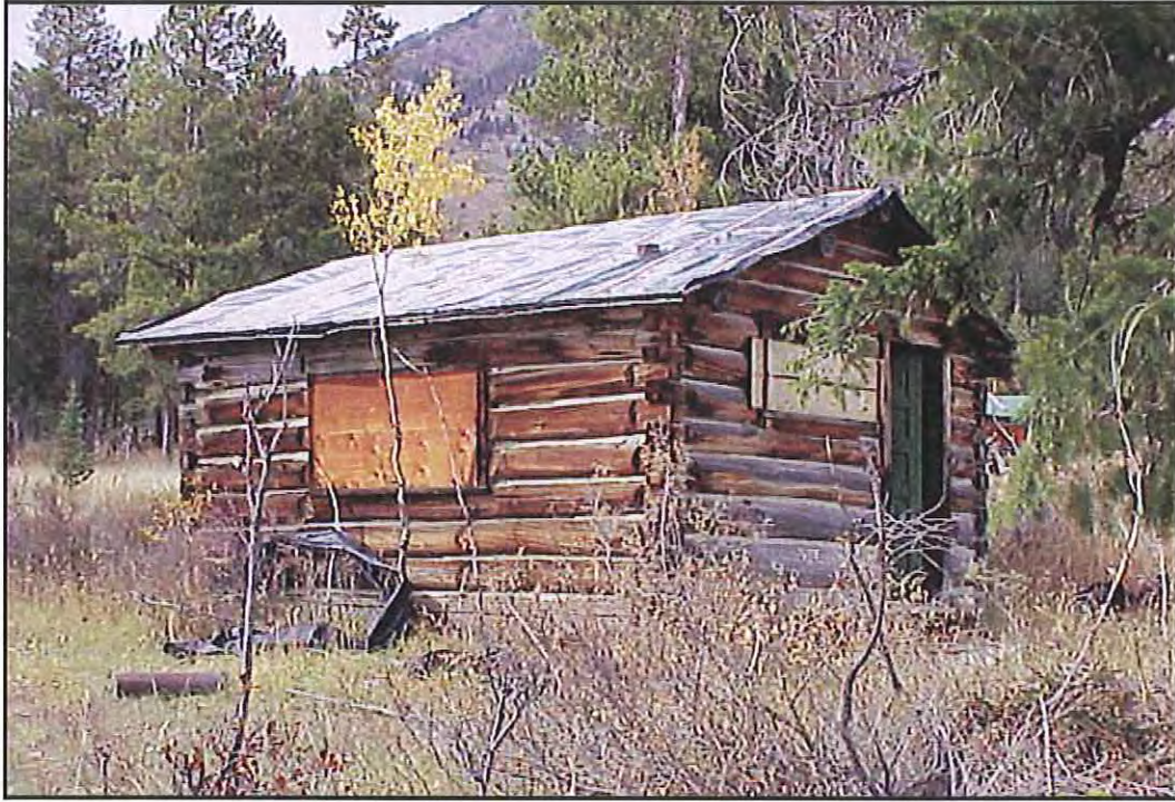
Figure 41. South and east walls of HS-1157, Cabin 12. Source: A&E Architects, 2004.
